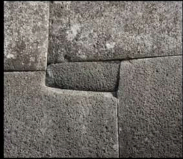
AHU VINAPU, EASTER ISLAND
