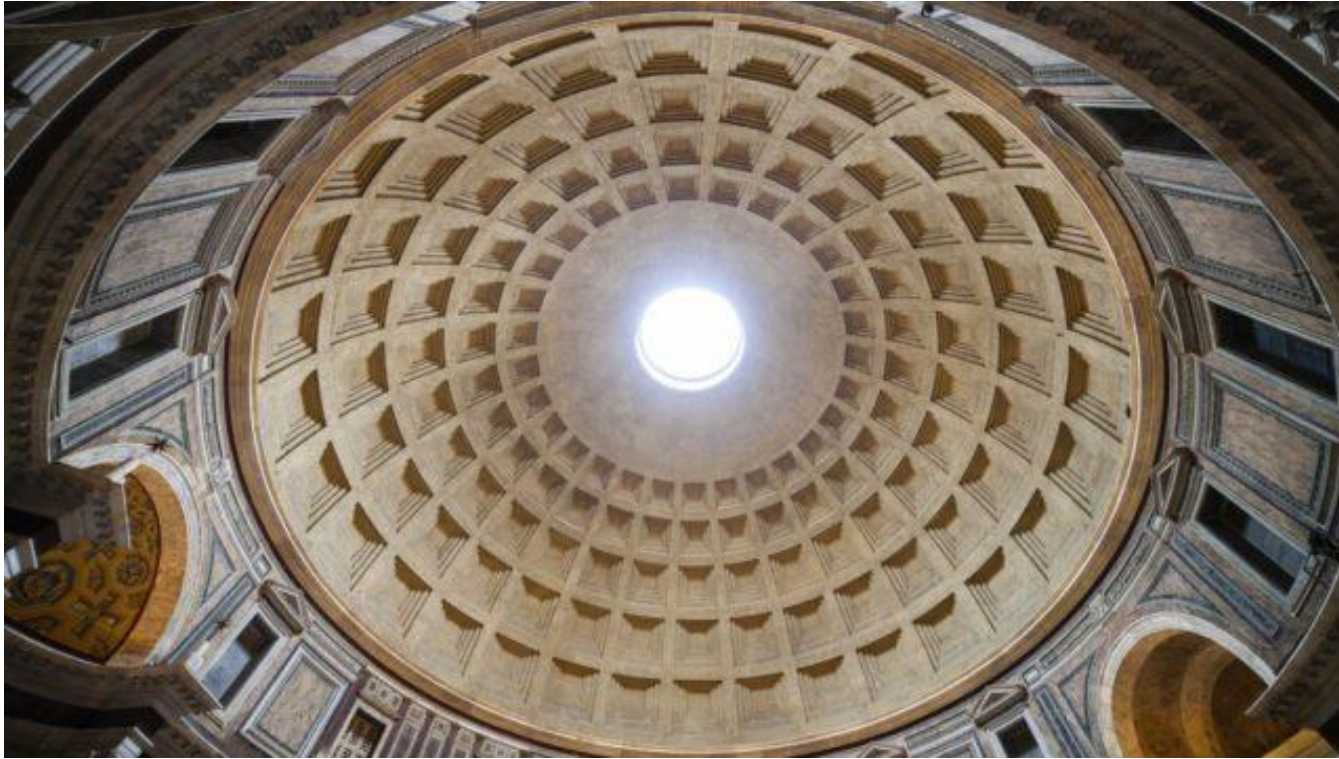
The oculus of the Pantheon of Rome, the world's biggest unreinforced concrete dome.
