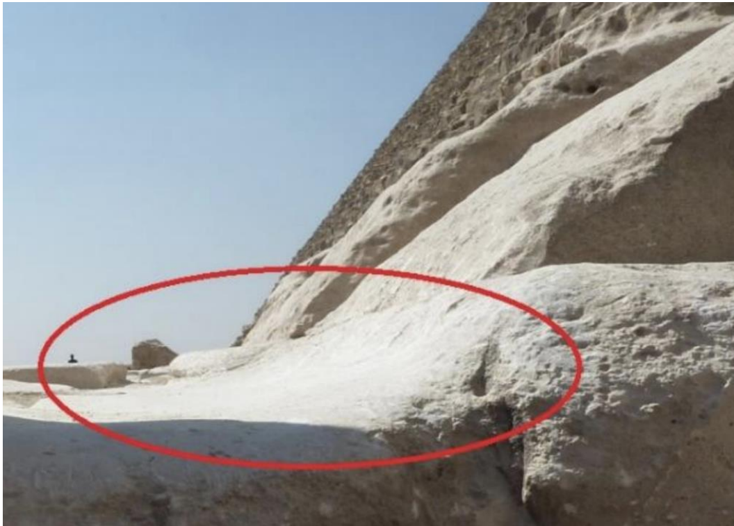
Uniform erosion on limestone rock.
