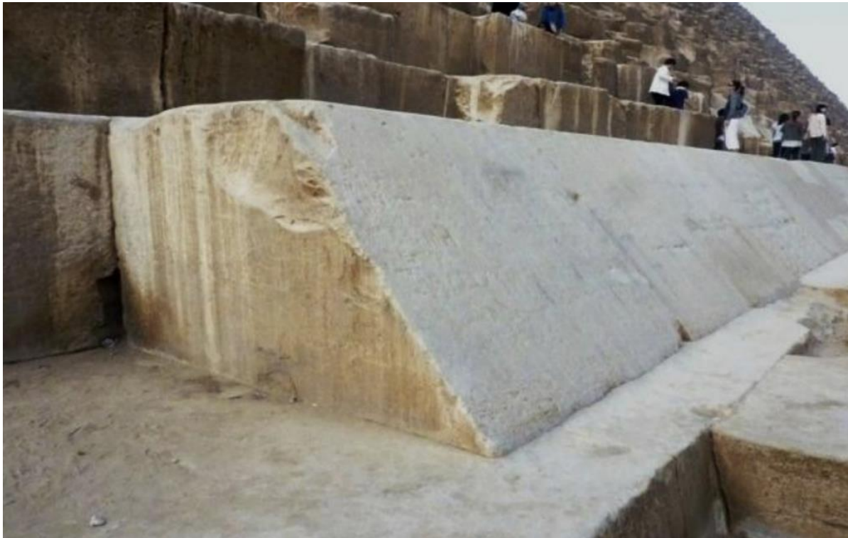
Base of Akhet Khufu with the few remaining limestone blocks of the cladding.
